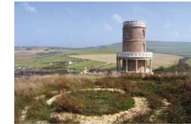
© The Landmark Trust. Clavell Tower was relocated 20m behind the original site in 2006 to secure its future.
