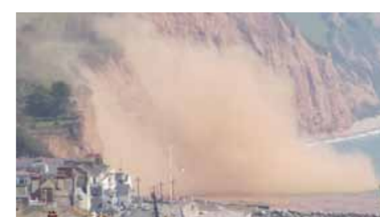
© Richard Gosling. Rockfall at Pennington Point, Sidmouth
